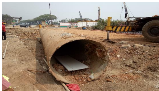
Gambar 3. Casing Tiang Eksisting Ø1,20 m
